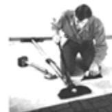
Use a mechanical device to replace knee/hand hammering
