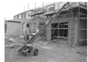
Use specially designed equipment to reduce repetitive handling/carrying
