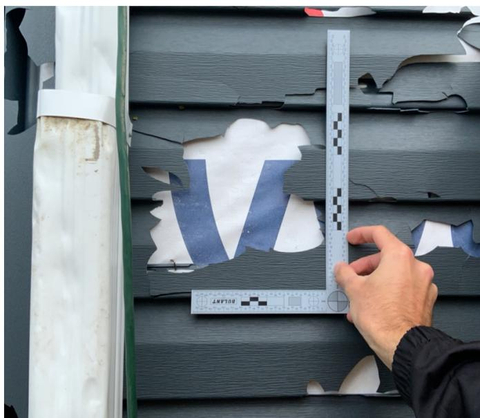
Figure 6: NHP team member holding a reference object to hail damage to residential siding.
